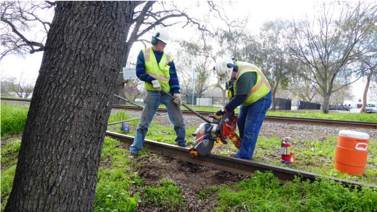
Steve uses a shovel as a spark-arrestor as Mike F. cuts into the rail with the rail-saw
