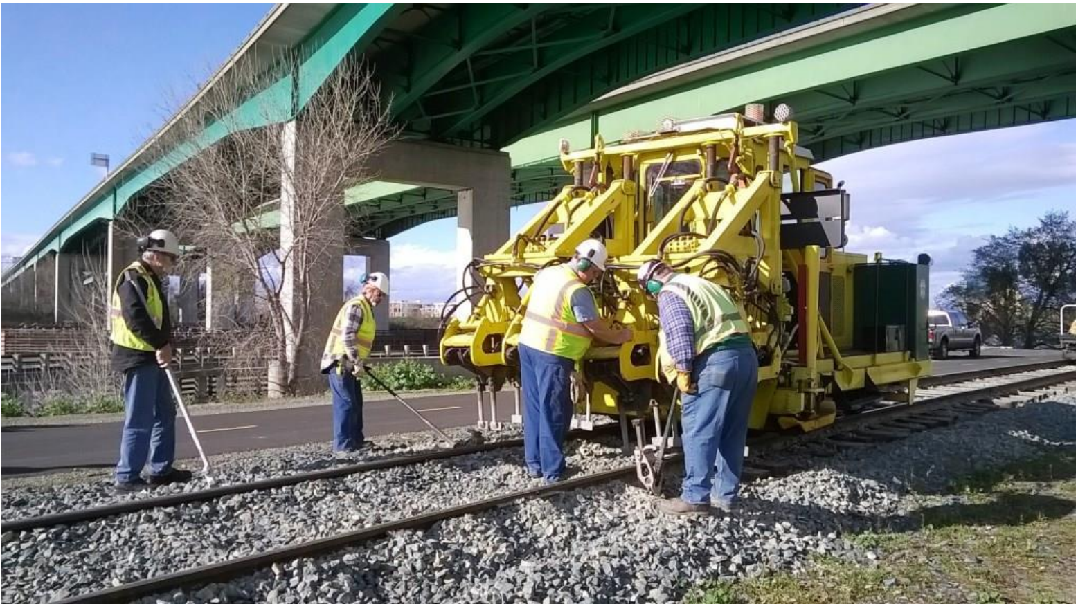
The Team works with Steve in the tamper to make sure the work-heads are "squeezing" rock under the ties
