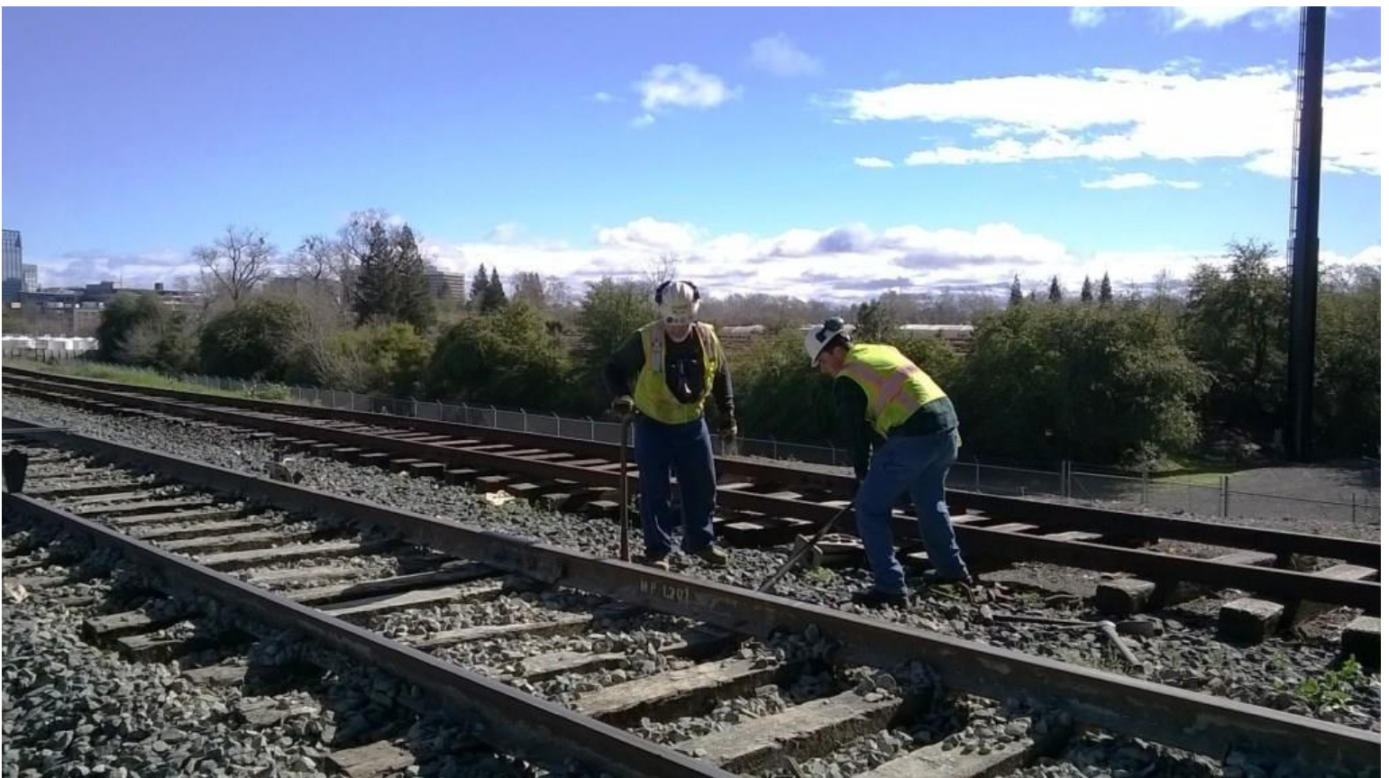
Mike F. and Weston nip-up a tie and hand tamp it
