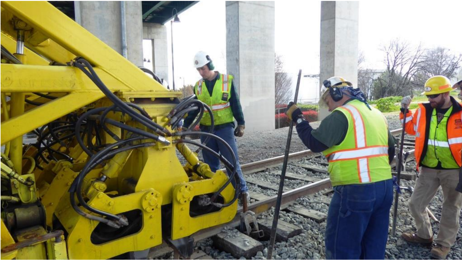
Weston guides the tamping from the ground
