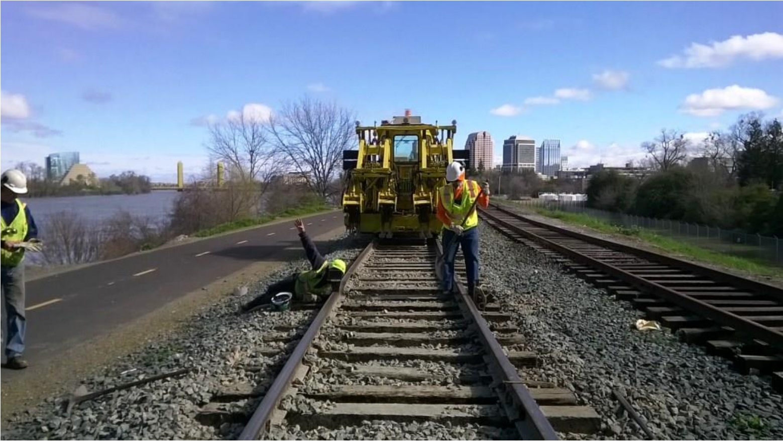
Joe, behind the "hound" giving the signal to the crew cranking on the jacks
