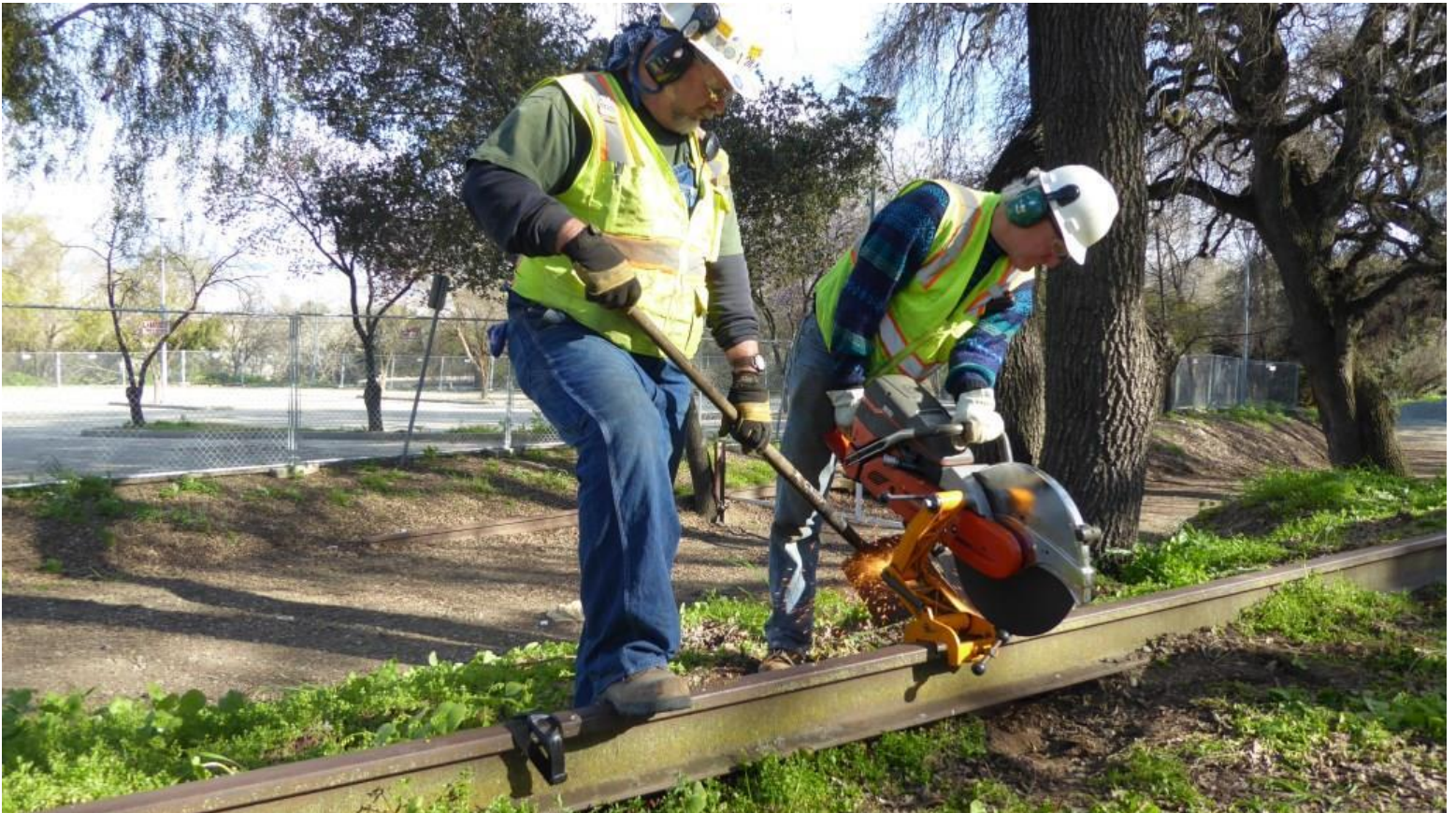
And now Steve cuts the second piece of rail for the Switch 19 frog as Mike F. holds the spark-arresting shovel
