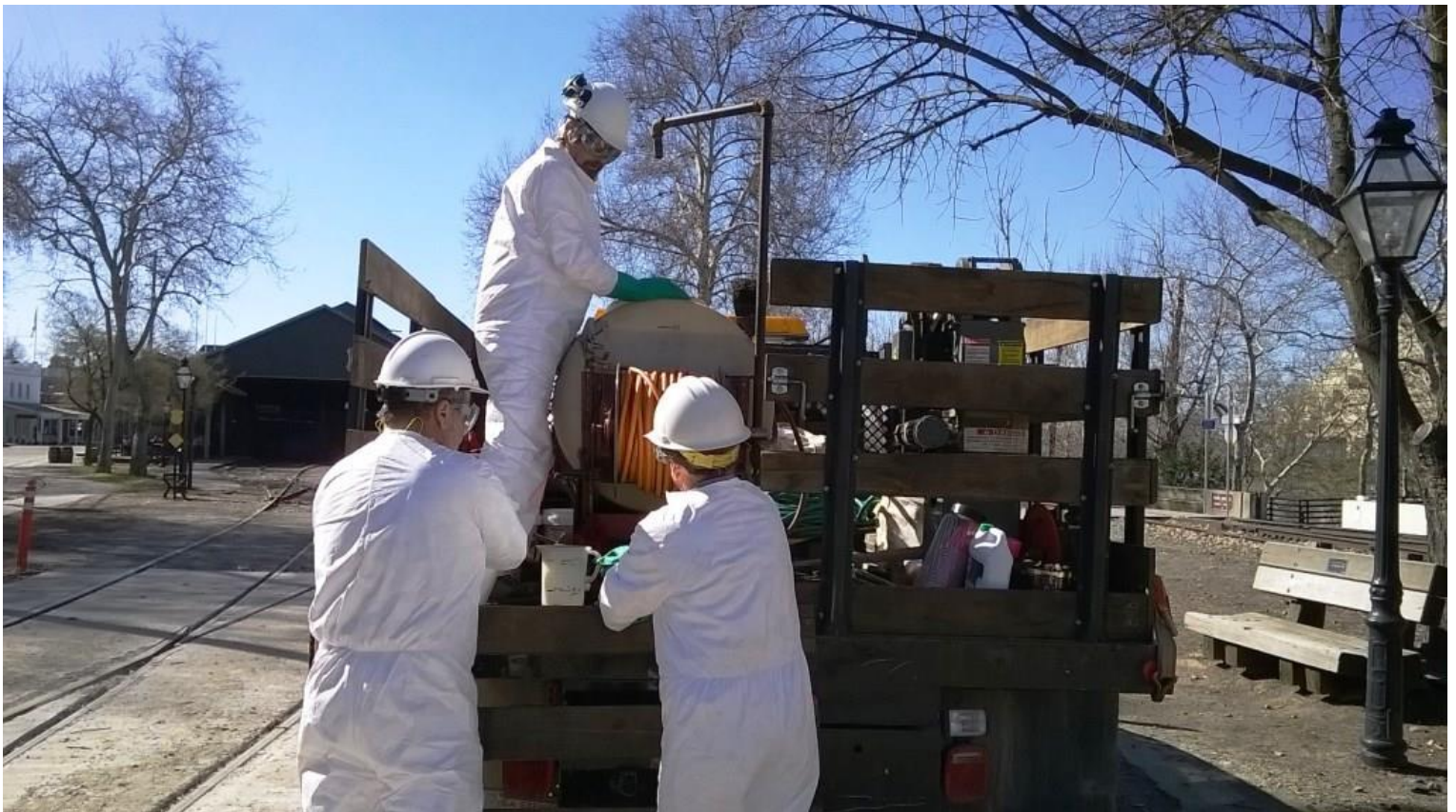
Steve, Ed, and Mike T. load the 65-gallon spray-rig into the truck
