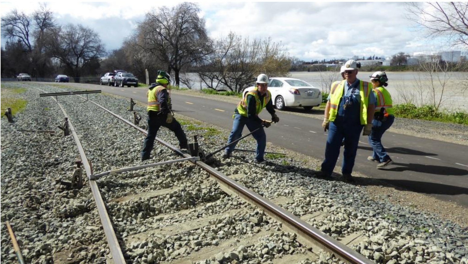
Weston follows Chris M.'s directions on how much to jack the track
