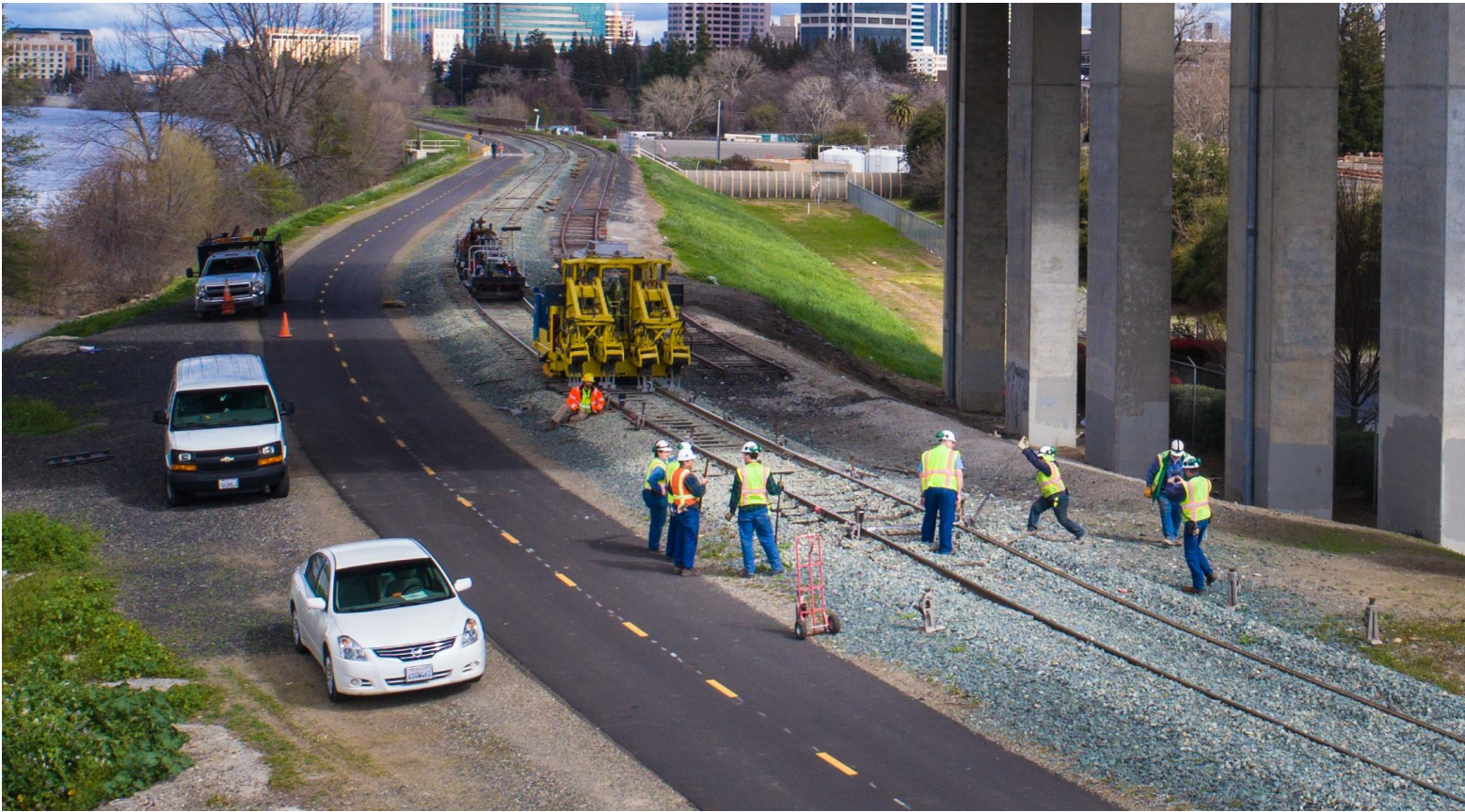
So, here are two views of the exact same moment from different perspectives of the MOW Team at work. Kelly captured this view of the track-raise in progress from his drone flying overhead...
