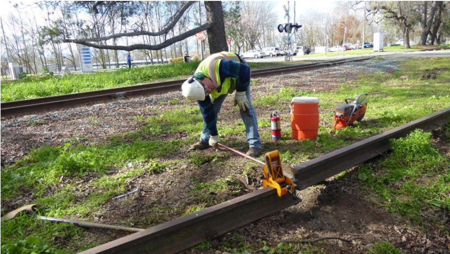
Steve uses a nipper-bar to snap the now cut rails apart
