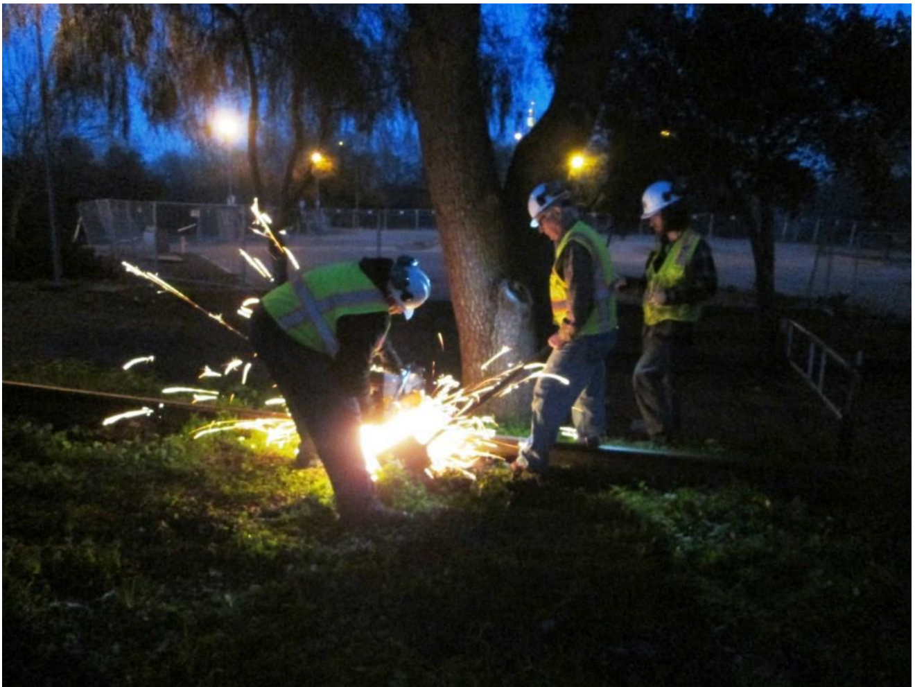
While the rail-saw was working, Harry starts cutting the rail as Mike W. uses a shovel as a spark arrester
