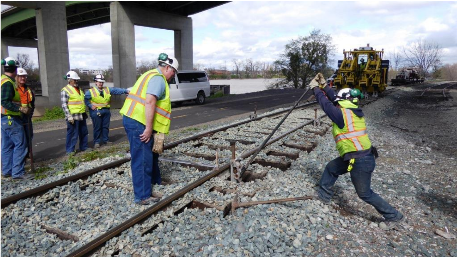
...While at the same moment, this photo of Chris C. and Joe leveling the track was taken from the ground
