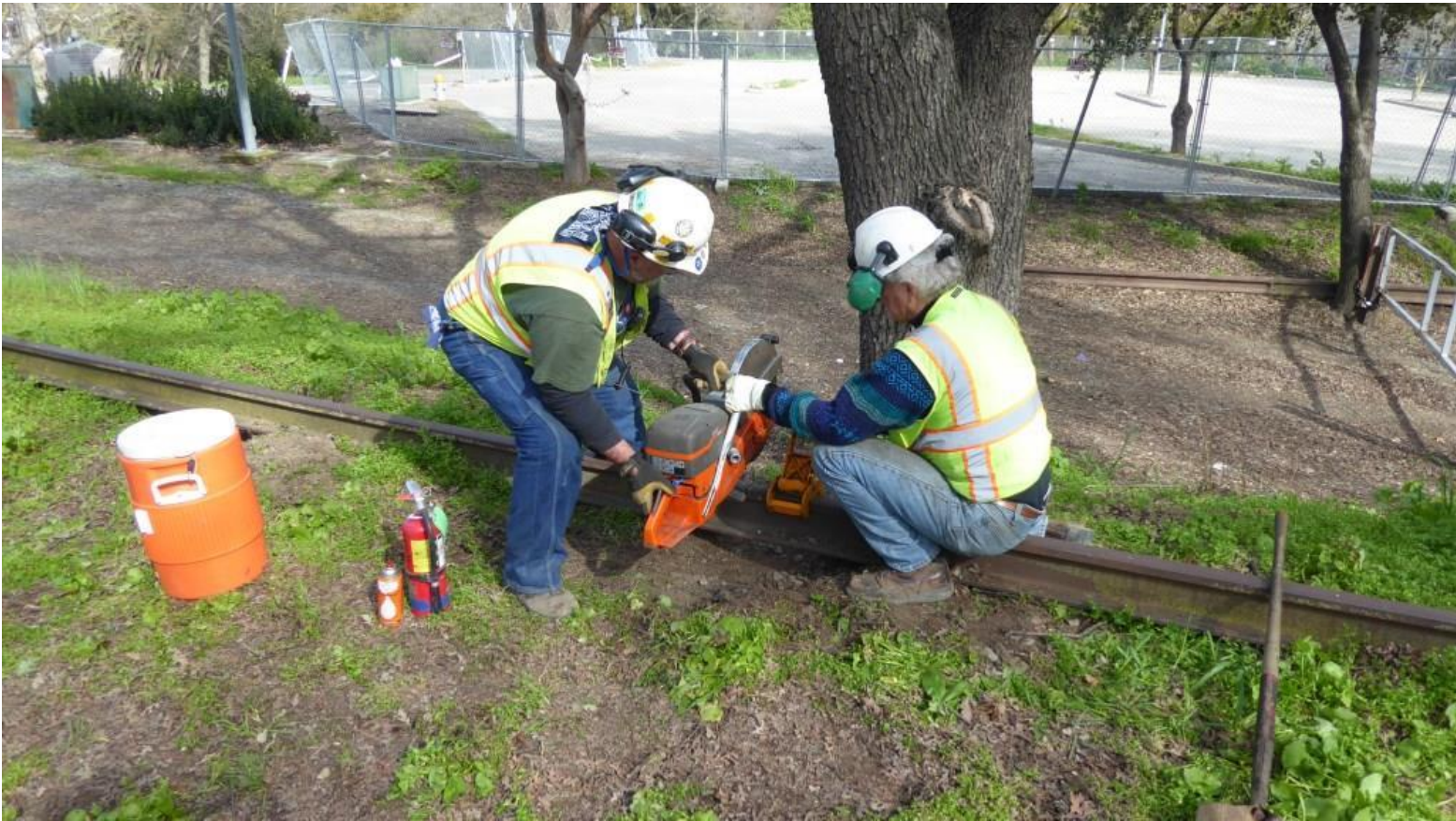
Mike F. and Steve set up the rail-saw on the spare stick of 110-pound rail to be cut for use in the Switch 19 frog
