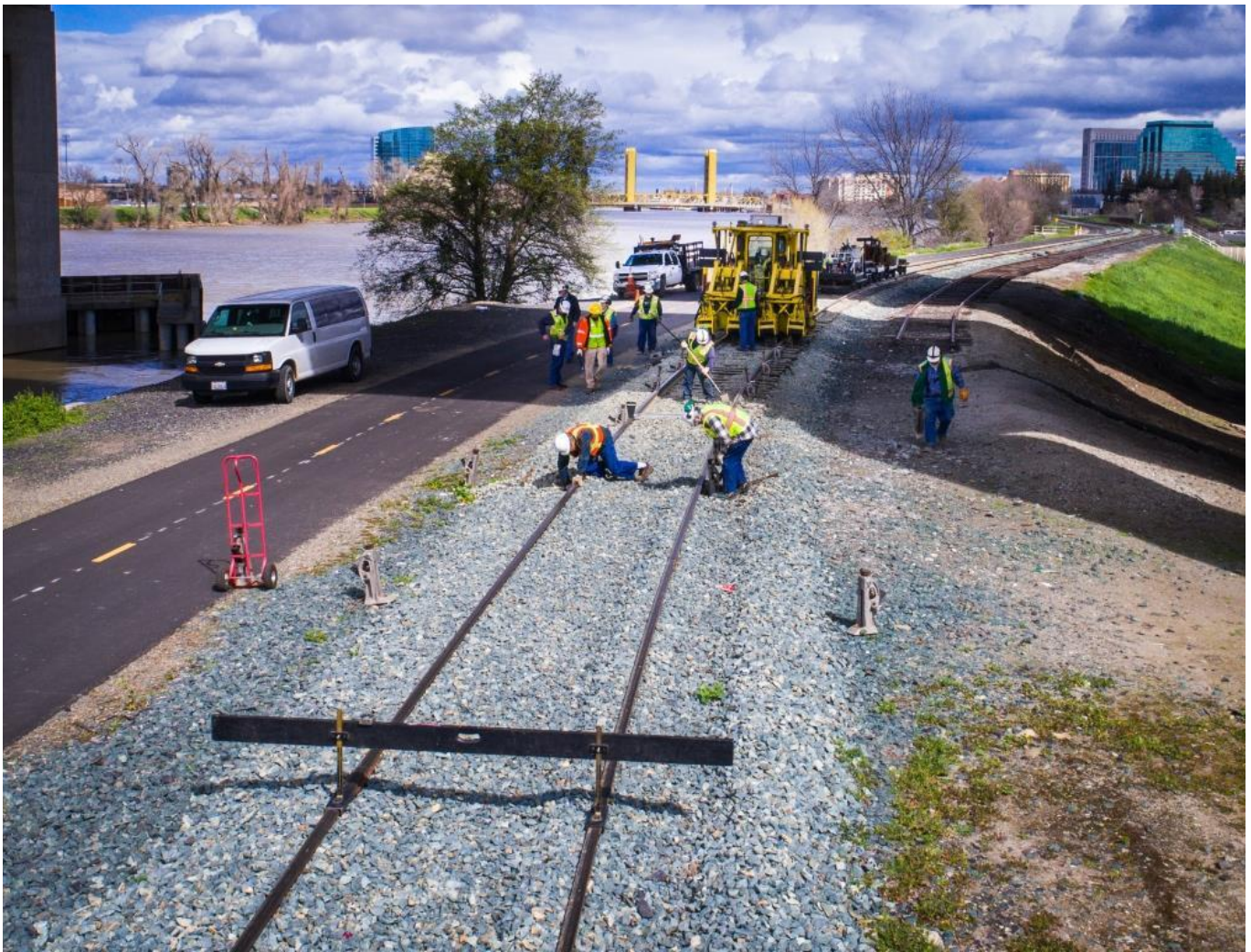
Another view from the drone showing the area being raised – from the spot-board in the foreground to the tamper in back
