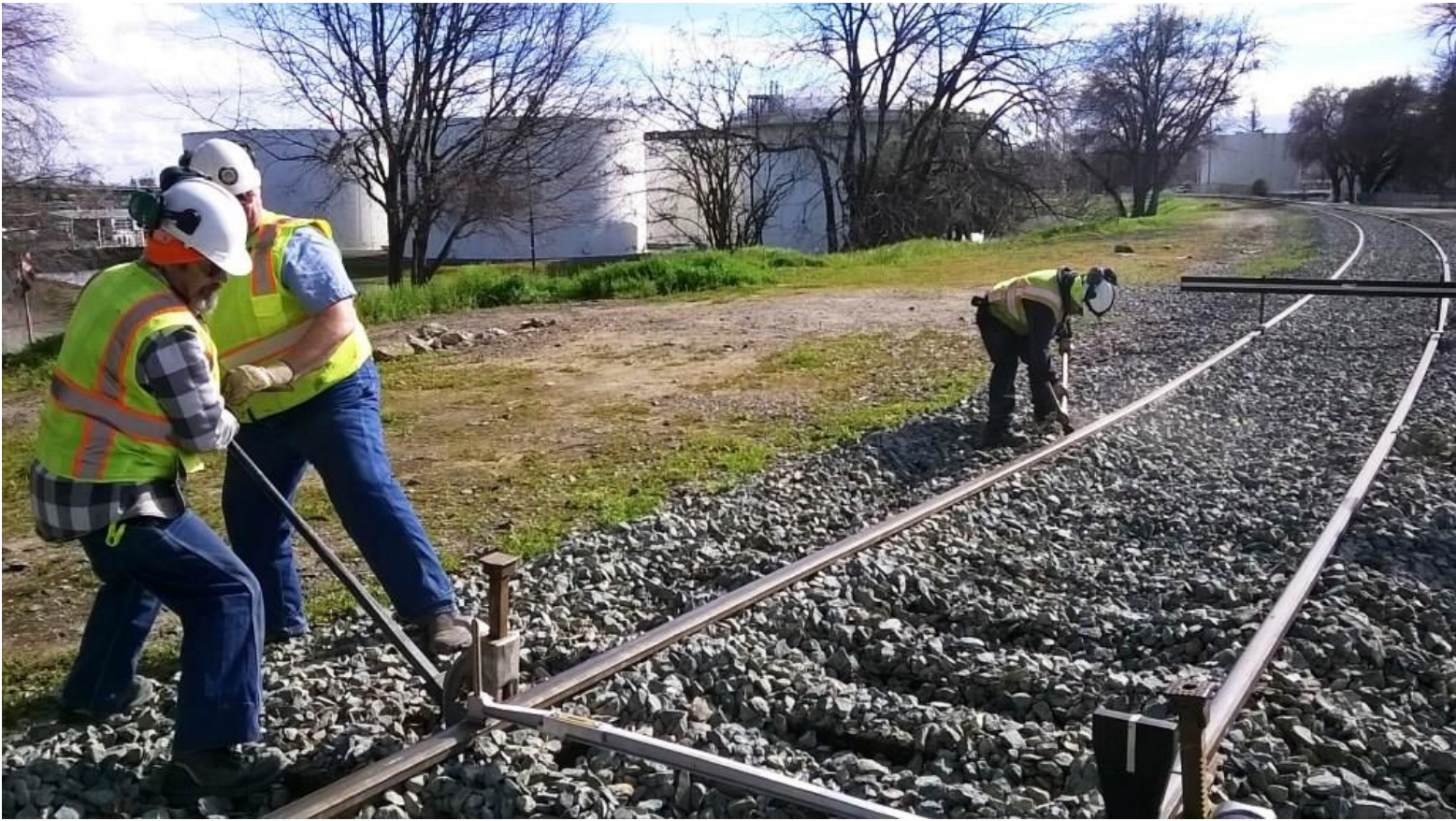
Chris and Ed combine forces to raise the east rail level with the west
